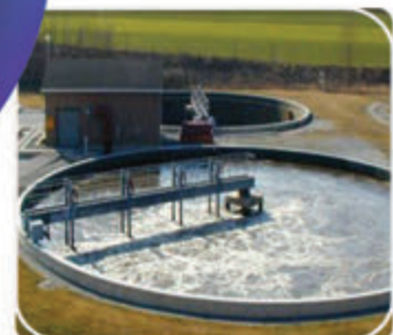
Industrial Wastewater Treatment Sewage
