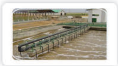
Wastewater Treatment Sewage
